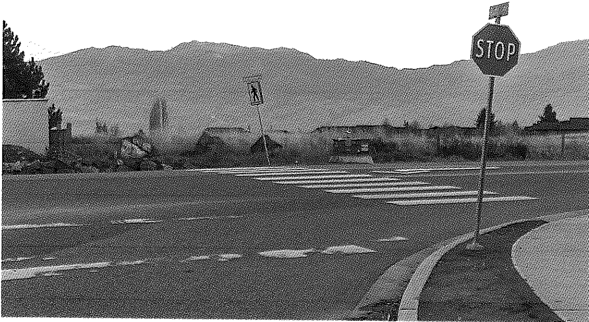
photo 2. Looking eastward, across Carrington from Butt . No overhead lighting for the crosswalk.
